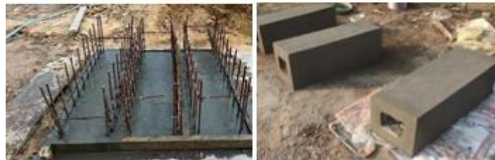
Fig.3 : RC Beam Casting
