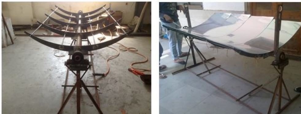
Fig 2 and 3 Fabrication of parabolic trough concentrator: Frame and Surface
