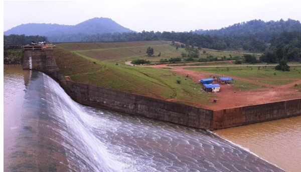
Fig-3: Pictorial view of Spillway of Paralkot dam
