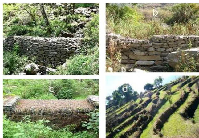
Figure: 3 Water recharge structures constructed in the study area (check dams and contour trenches)
