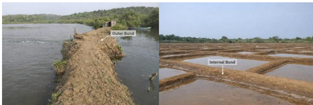
Figure 2: Bund structures of the Khazan system
